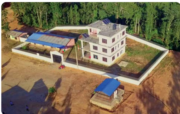
1 kWp solar panels gracing the rooftop of the Ward Office in Panchapuri Municipality-2, Surkhet.
