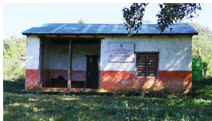
Community Health Post in Puchma Village, Chakune Municipality, Surkhet.
