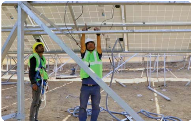
Installations taking place in Thosnekhola RSDWP, Lalitpur district.
