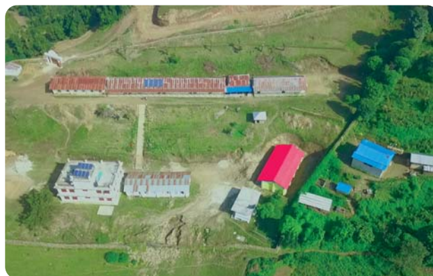
Sarwaswoti Secondary School in Yuoo Village, Aamchowk 2, Bhojpur, now energized with ISPS.
