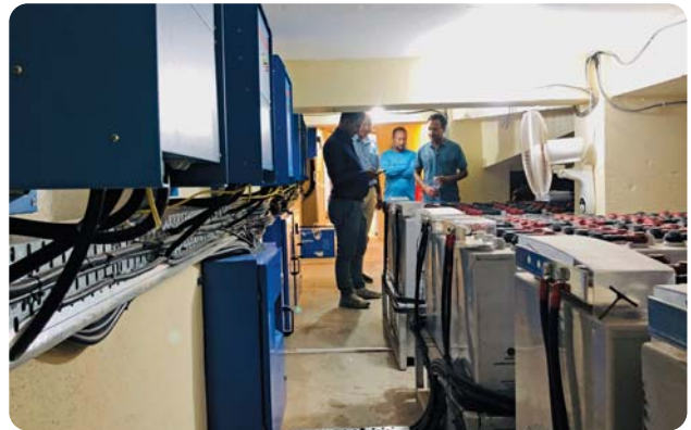
Testing and Commissioning of the Large scale ISPS at Gorkha Hospital in Gorkha Municipality-6.
