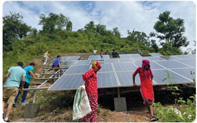
Community members of Chainpur Municipality in Sankhuwasabha actively engaging in the execution of the Piliwakhola Rural Solar Drinking Water Project.
