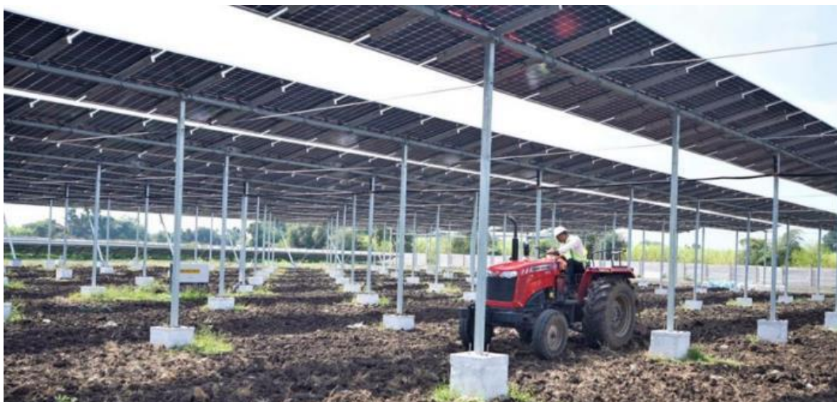
Figure 18: Tractor tilling under a 1.5 MW agrivoltaics power plant in Maharashtra, India 156
