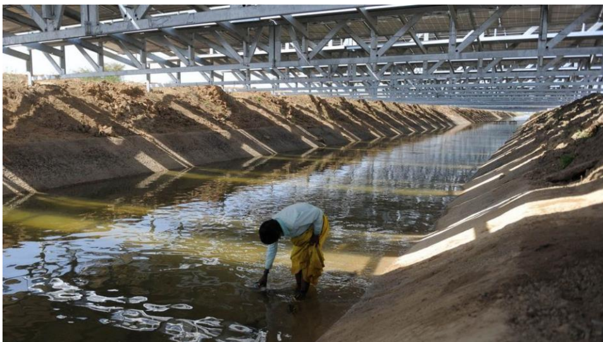
Figure 20: Canal-top solar in Gujarat 163
