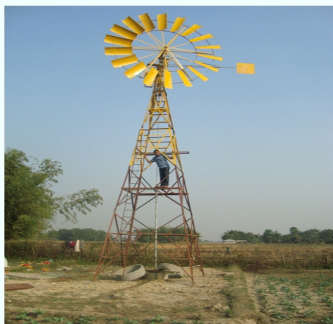
Figure: - Wind pumping system at Vahauda VDC, Morang district
