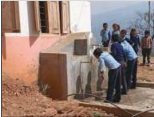
Piluwa Khola Rural Solar Drinkg Watersupply Project at Chainpur Municipality-10, Sankhuwasabha
