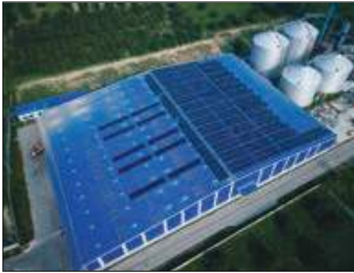
Solar Rooftop installed in Bhudeo Khadya Udhyog with support from AEPC/NREP
