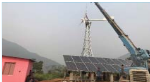
Figure 24: Installation of wind-solar hybrid system in Hariharpur Gadhi, Sindhuli
