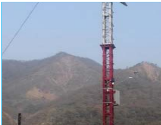
Figure 22: Data logger for wind energy
