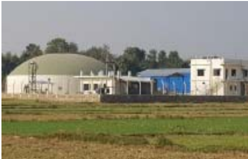
Figure 19: A large biogas plant installed in Nawalparasi district
