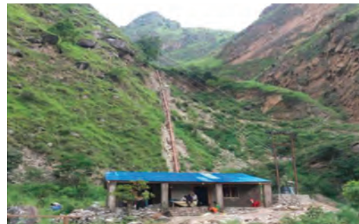
Figure 10: Powerhouse at Lagagad MHP, Kalikot, 85 kw, Pachaljharana
