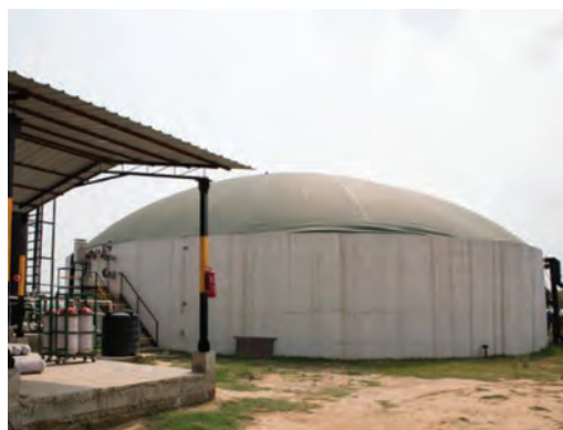
Figure 18: Envipower Nepal Energy & Fertilizer company, Bhairahawa 3700 m 3 biogas Plant for Bio-CNG Bottling and sale
