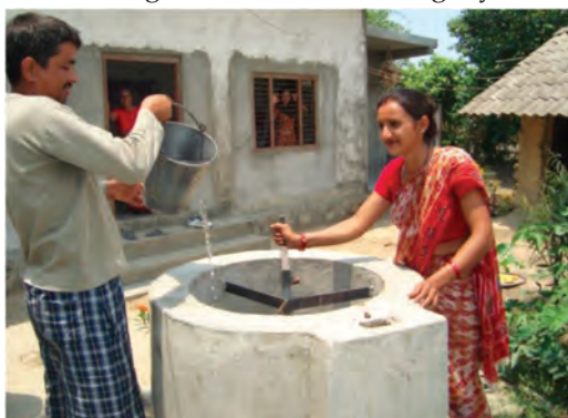
Figure 16: Feeding cow dung in biogas digester
