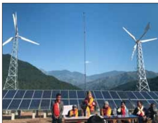
Figure 18: Solar Wind Mini Grid at Chisapani, Sindhuli
