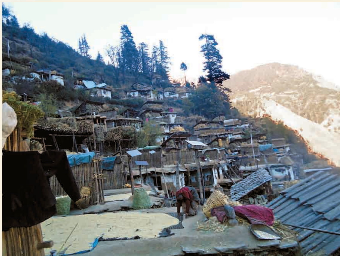
A cluster of 50 houses in Dolpa have installed Solar Home Systems.
