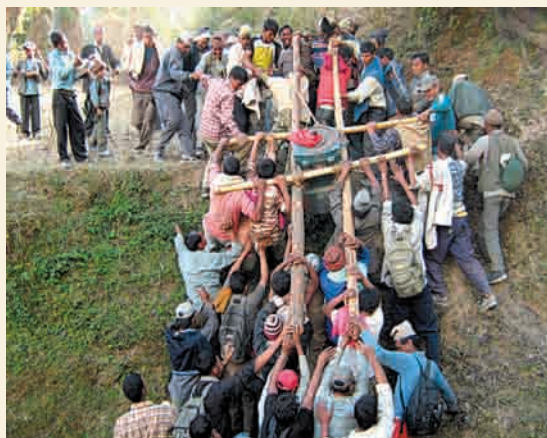
Community members of the Sain Gad MHVEP, Bajhang are transporting a 50 kVA generator.
