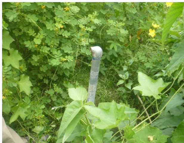
Both of us are Plant: Biogas Plant Covered by Green Plants
