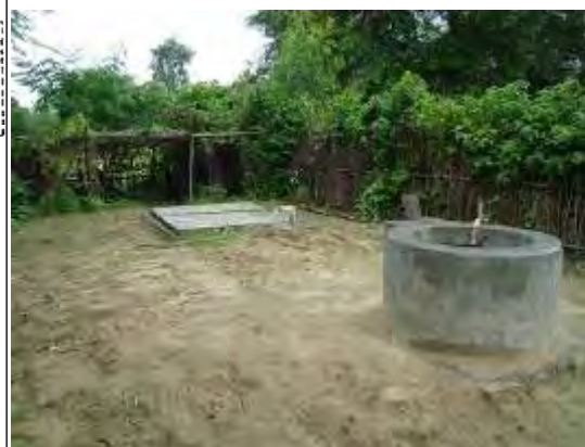
Fig: Biogas Digester in Operation
