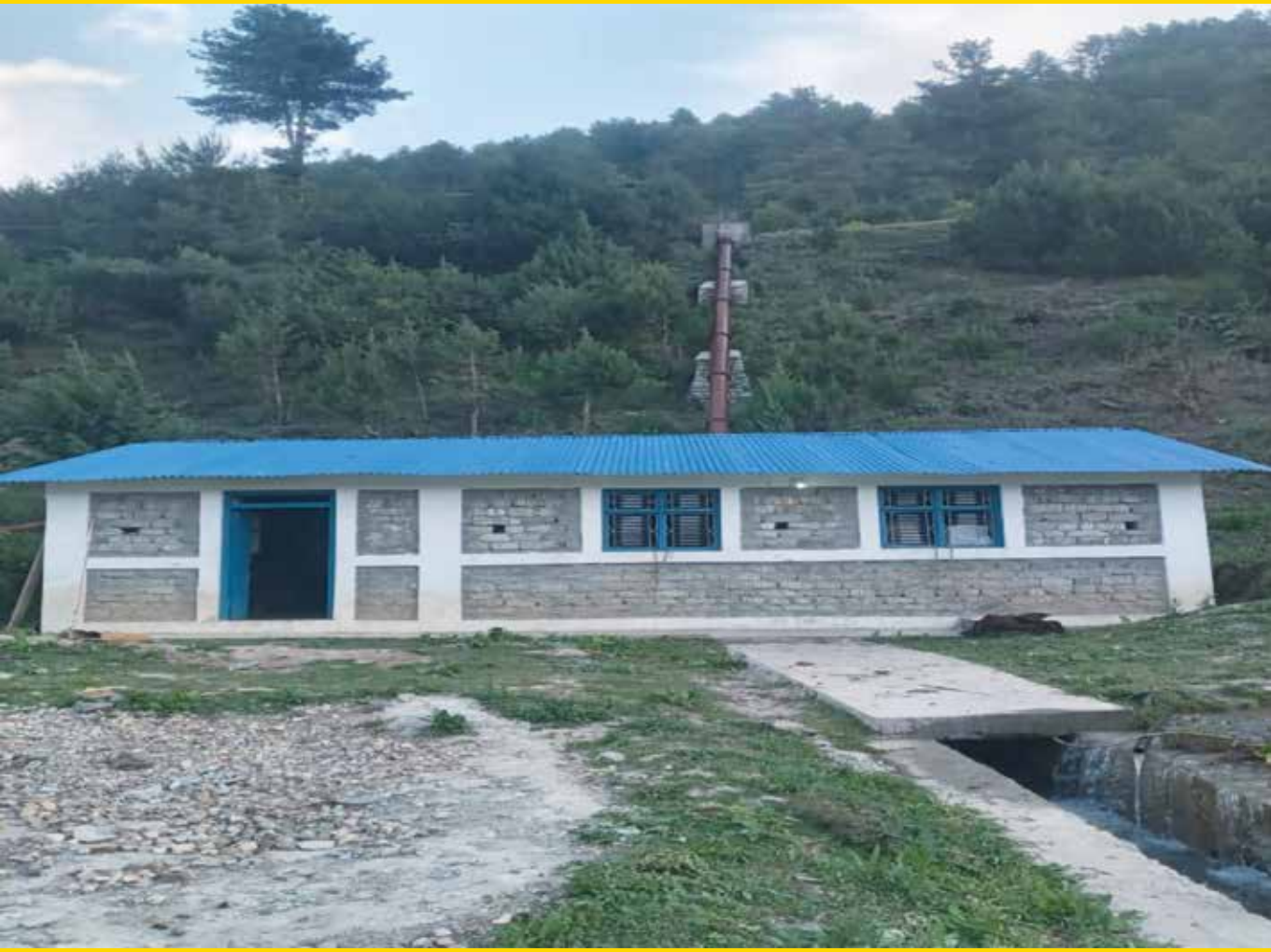
Dhorpatan Bhuji Khola MHP (60 kW) at Dhorpatan Municipality-9, Baglung
