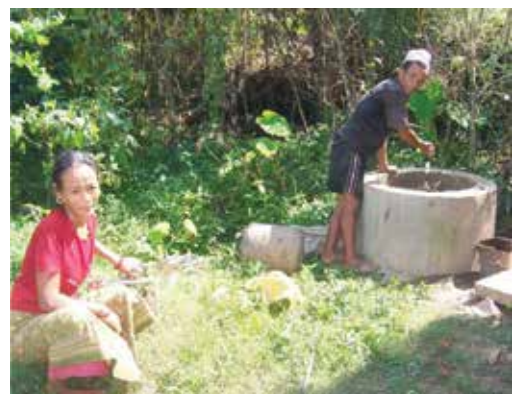
Figure 15: Domestic Biogas Plant installation
