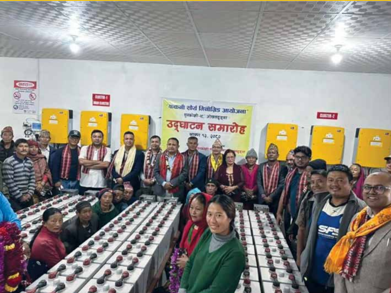
Mr. Dinesh Kumar Ghimire, Secretary (Energy), Ministry of Energy, Water Resources and Irrigation, together with relevant officials and local people during inauguration of Sunkoshi Kakani Solar Minigrid Project (70 kWp) at Sunkoshi Rural Municipality, Okhaldhunga
